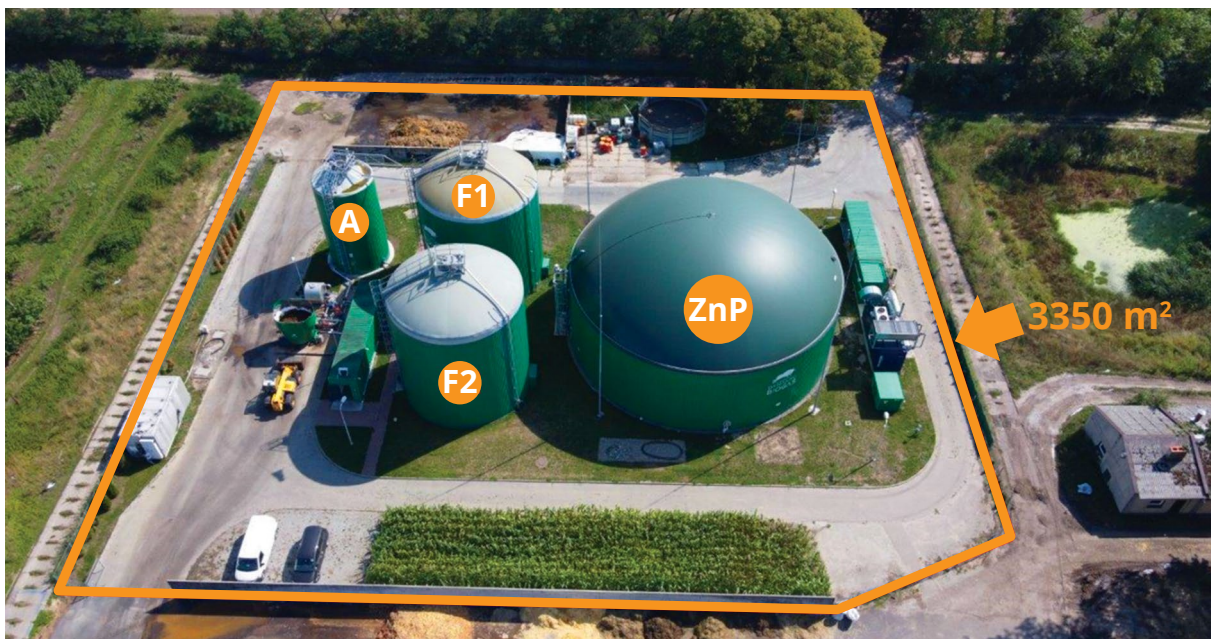
FIG. 16. View of the biogas plant (biomethane production potential of 2.1 million m 3 /year) at the UPP farm in Przybroda; A - biotechnology accelerator (250 m 3 volume), F1, F2 - fermenters (2 times 870 m 3 ), ZnP - digestate tank (3600 m 3 )
